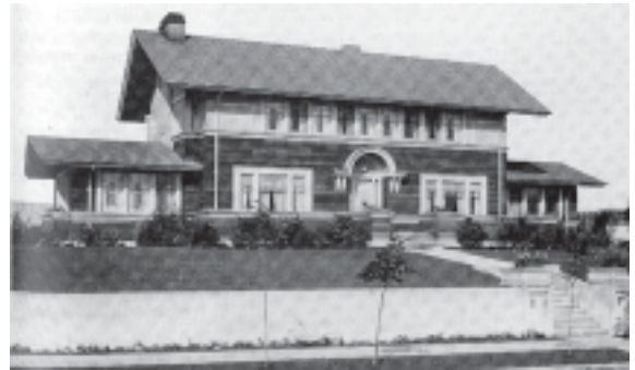
Queen Anne's now-demolished Black House
